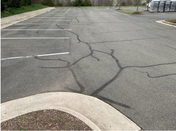
Asphalt pavement at clubhouse parking area
