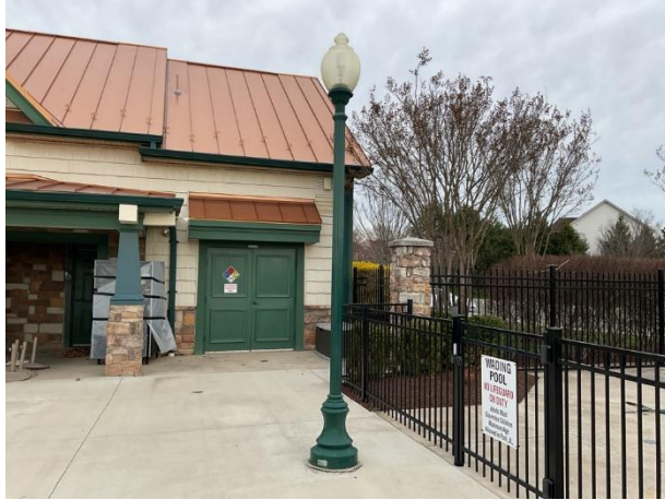
Light pole and fixture overview
