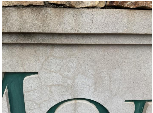
Sign cracks
