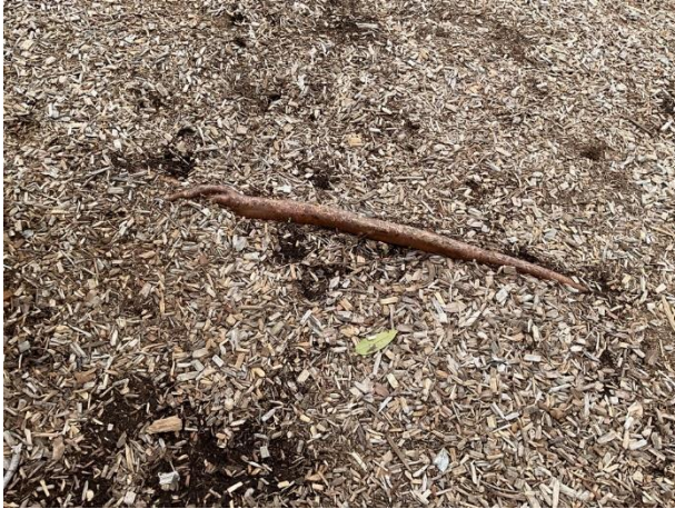
Exposed tree root at clubhouse playground
