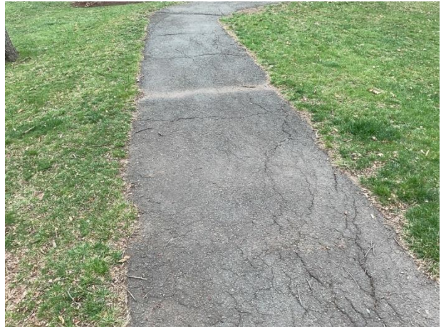
Pavement cracks
