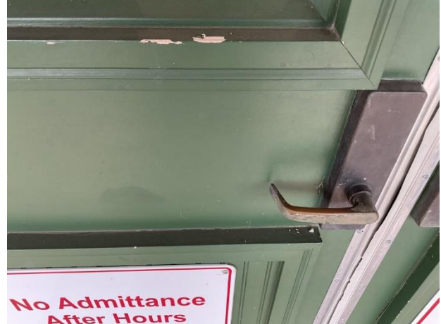
Finish deterioration
