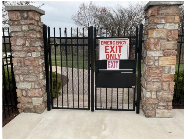
Pool gate overview
