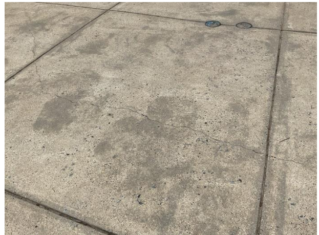
Concrete crack
