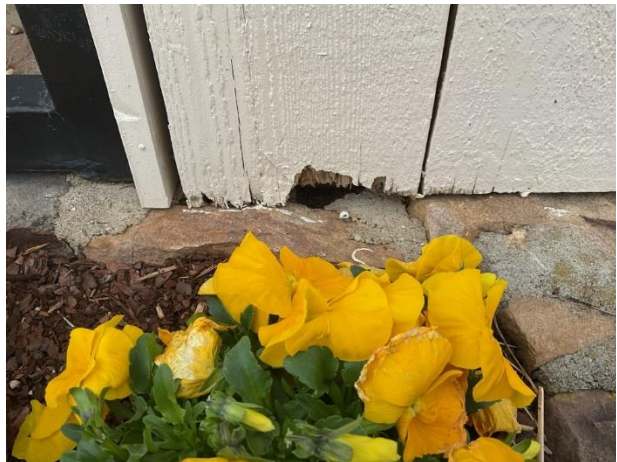
Trim deterioration
