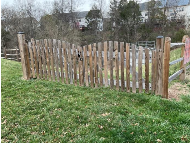
Gate at split rail fence
