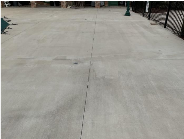
Pool deck overview
