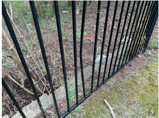
Damaged pickets
