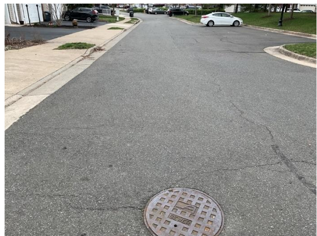
Asphalt pavement street at townhomes overview
