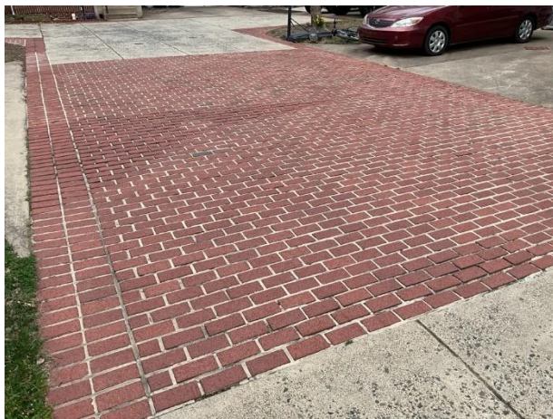
Masonry pavers overview
