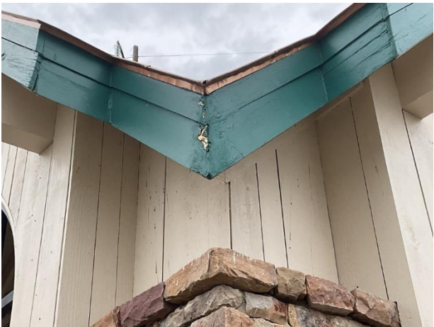
Trim deterioration
