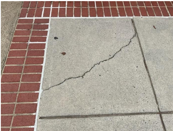
Concrete crack
