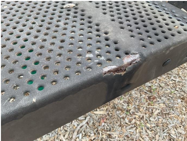
Finish deterioration and rust at clubhouse playground
