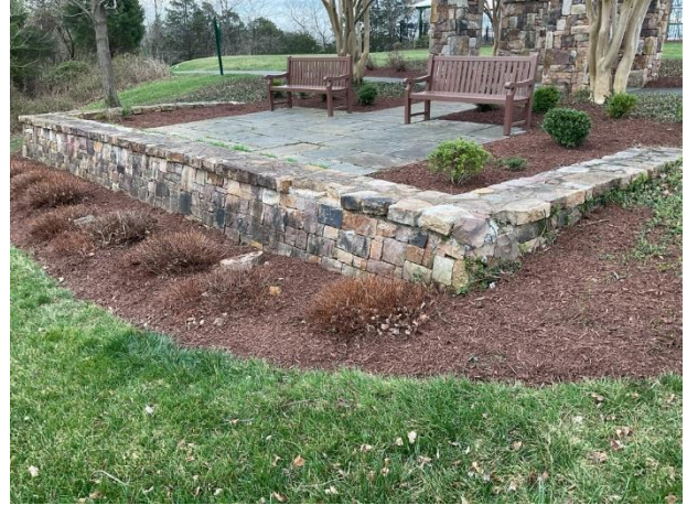
Stone retaining wall overview
