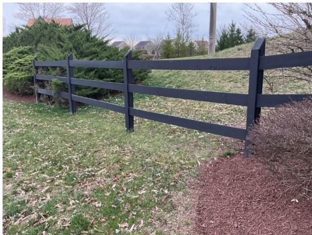
Open rail wood fence overview
