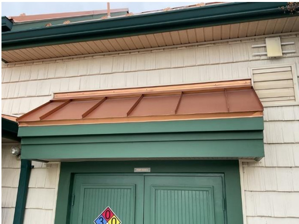
Metal roof overview
