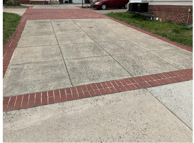
Concrete driveway overview
