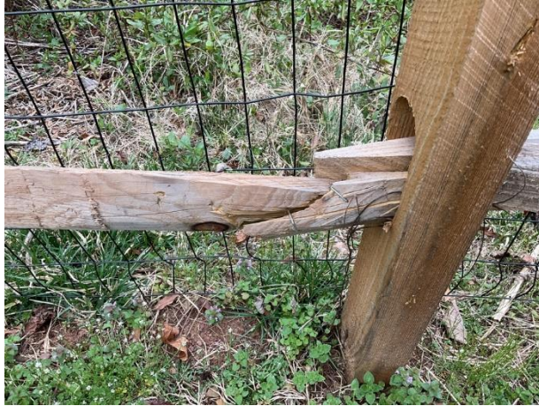
Broken rail at split rail fence
