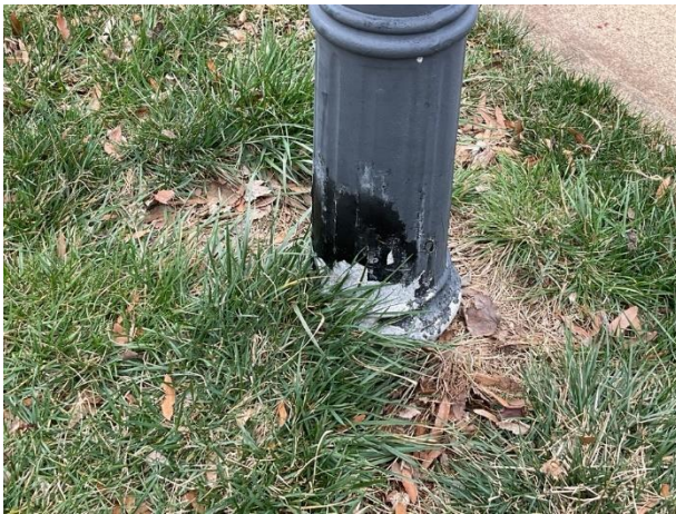
Finish deterioration
