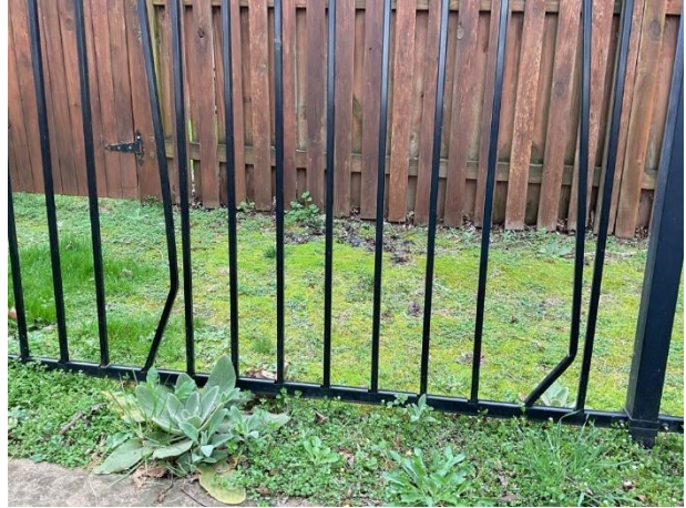
Damaged pickets
