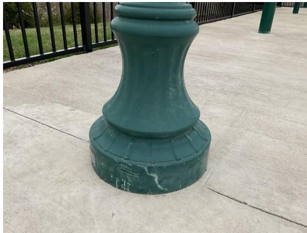
Finish deterioration
