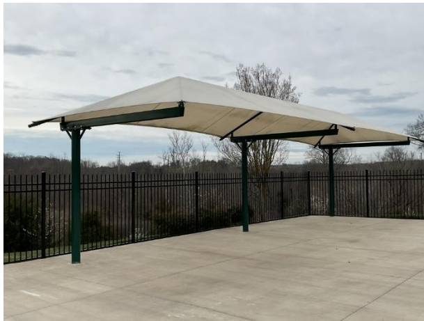
Shade structure overview
