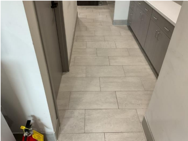
Tile floor coverings overview
