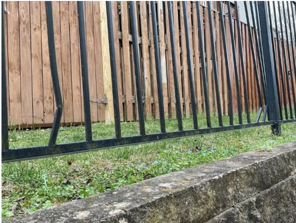
Damaged pickets
