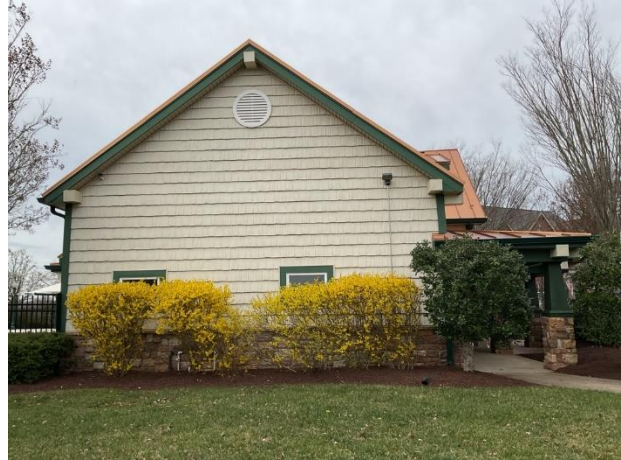
Clubhouse side elevation overview
