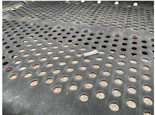
Finish deterioration and rust at clubhouse playground
