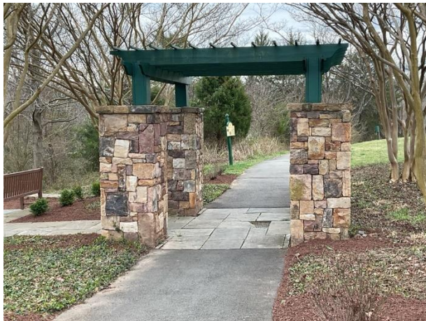
Pergola at clubhouse
