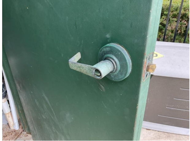
Corroded handle
