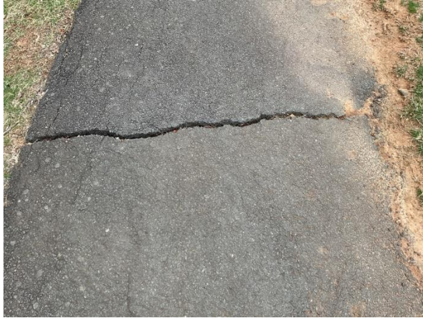
Pavement cracks
