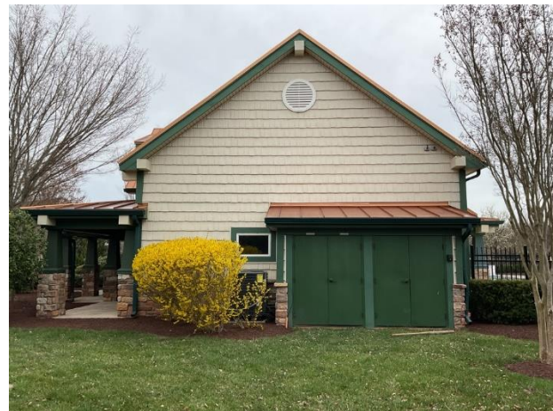
Clubhouse side elevation overview
