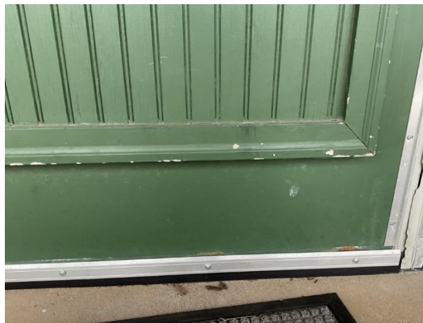
Finish deterioration
