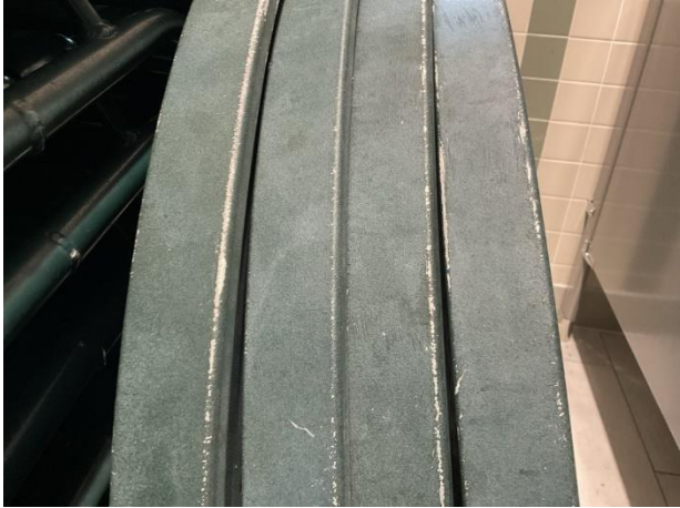
Finish deterioration
