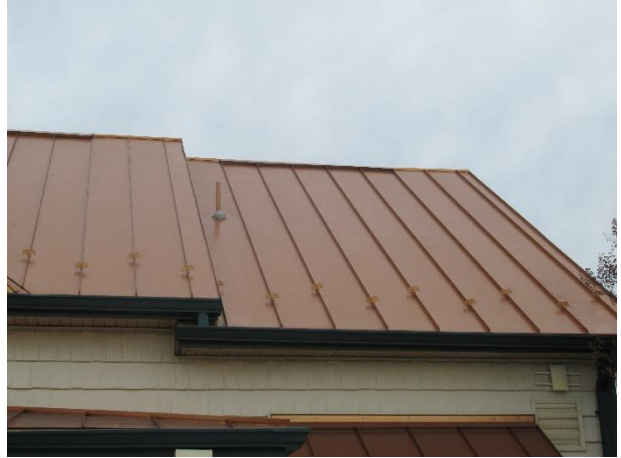
Metal roof assembly overview
