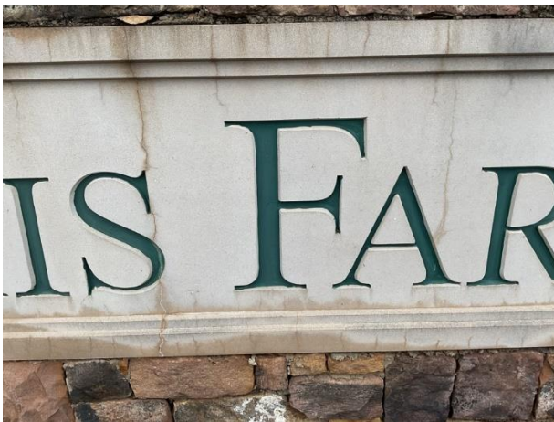
Sign cracks
