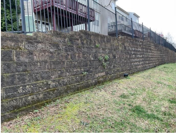
Masonry retaining wall overview
