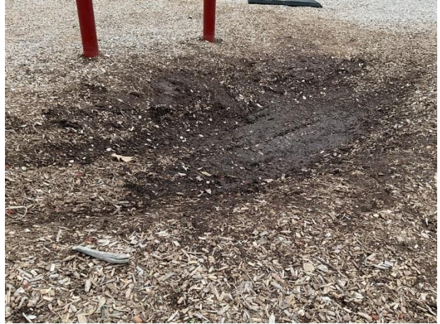
Mulch depletion at clubhouse playground
