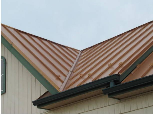
Metal roof assembly overview
