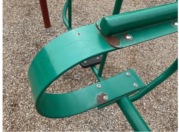
Finish deterioration and rust at clubhouse playground
