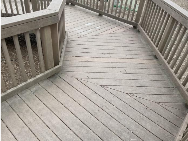
Deck boards overview
