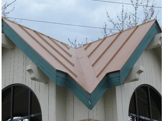
Metal roof overview
