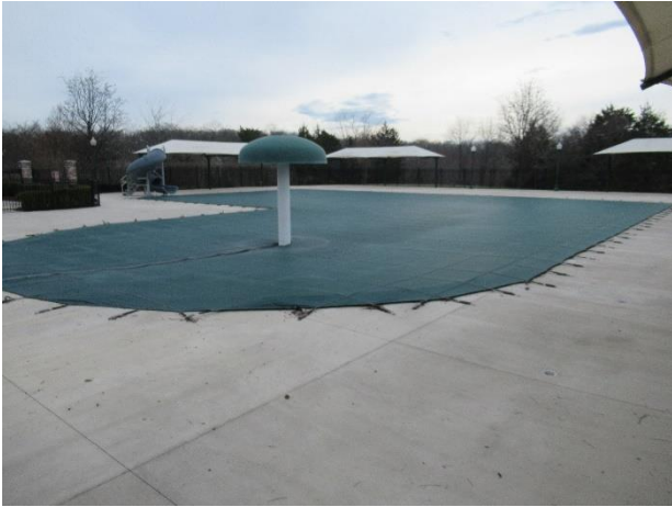
Main pool overview
