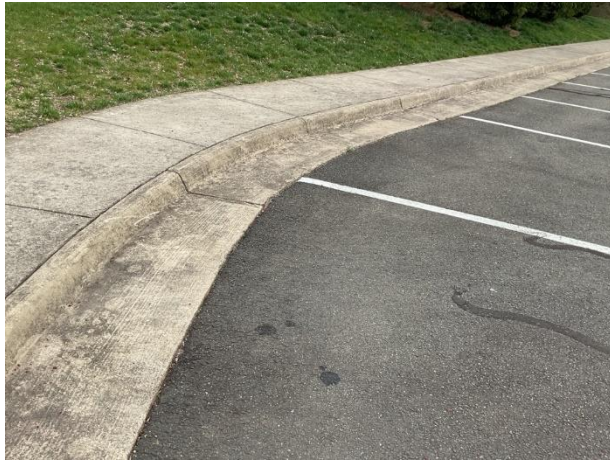
Curb and gutter overview
