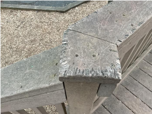
Railing deterioration
