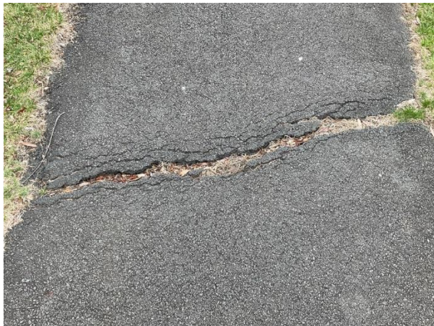
Pavement cracks
