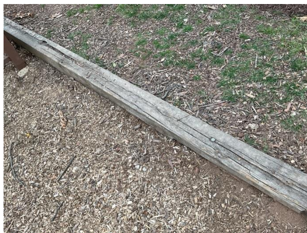
Wood split and deterioration at Parula Way playground
