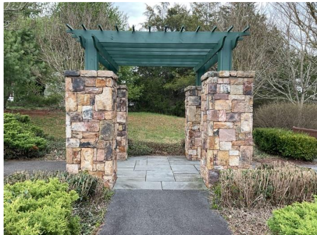
Pergola at Yellow Hammer Drive
