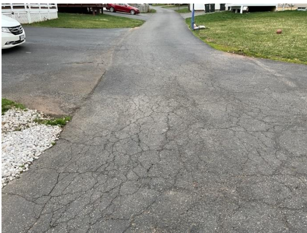
Asphalt pavement alley overview
