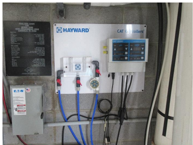
Automatic chlorinator
