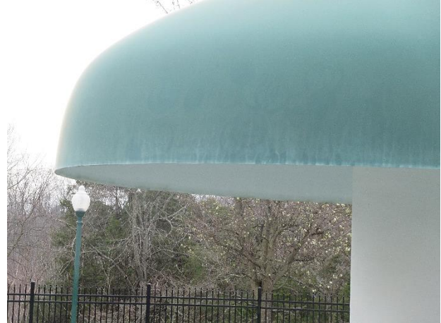
Finish deterioration
