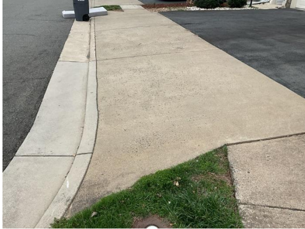
Concrete apron overview
