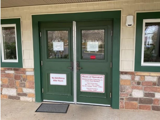
Entrance doors overview
