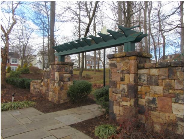
Arbor and masonry wall at Parula Park
