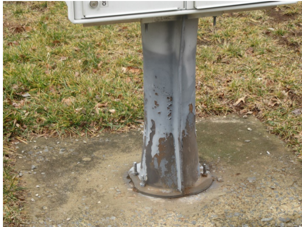
Mailbox station finish deterioration and fastener rust
