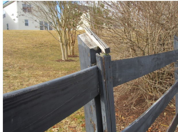
Open rail fence cracked picket
