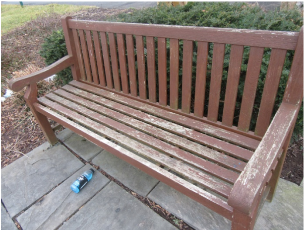
Site furniture; we note finish deterioration
