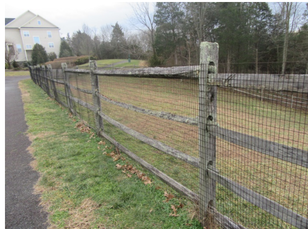
Split rail fence; we note organic growth
