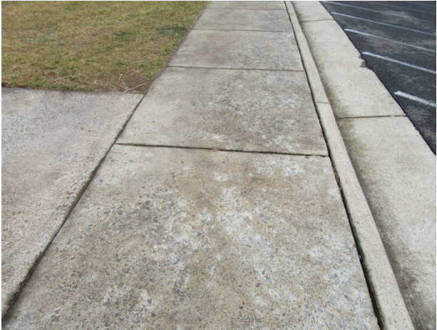
Sidewalk spall
