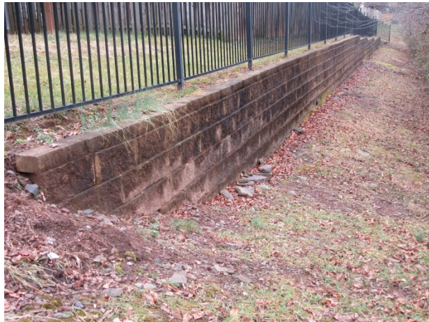
Masonry retaining wall
