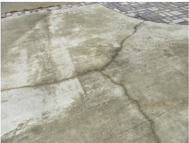
Deck cracks
