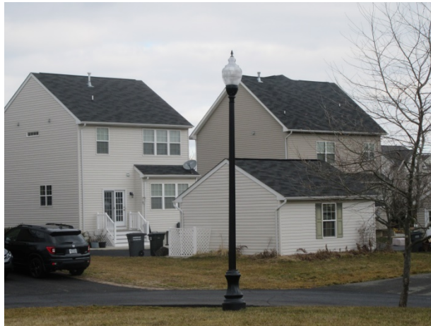
Light pole and fixture
