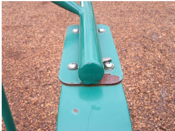
Rust at the clubhouse Playground equipment
