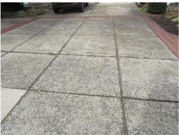
Concrete spall
