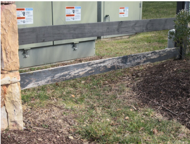
Open rail fence finish deterioration
