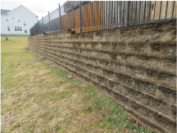
Masonry retaining wall
