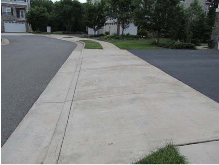
Concrete driveway apron
