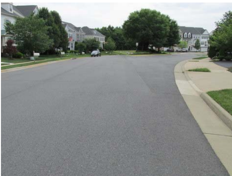
Asphalt pavement street at Catbird Drive
