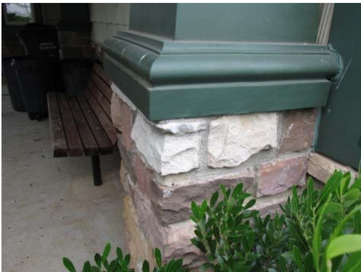
Masonry veneer at clubhouse
