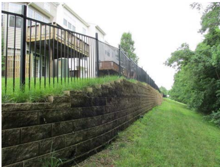
Masonry retaining wall
