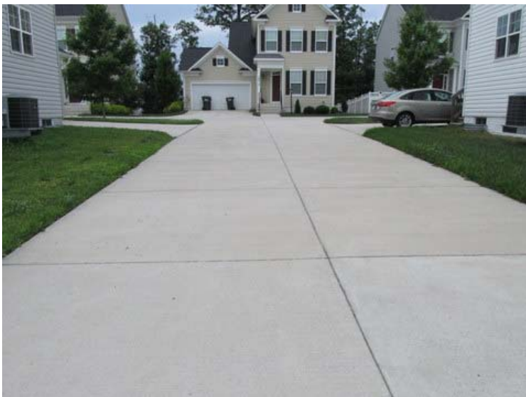
Concrete driveway at cluster homes
