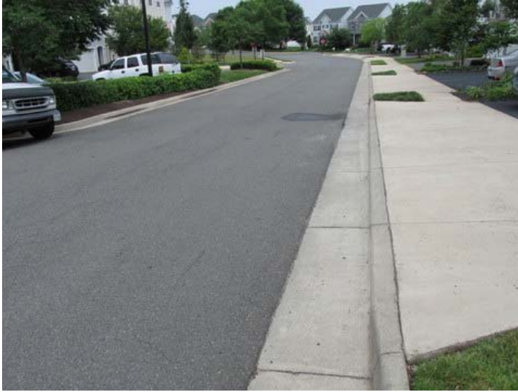
Asphalt pavement street at Catbird Drive
