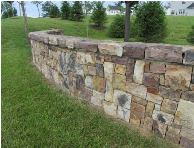
Masonry veneer at entrance
