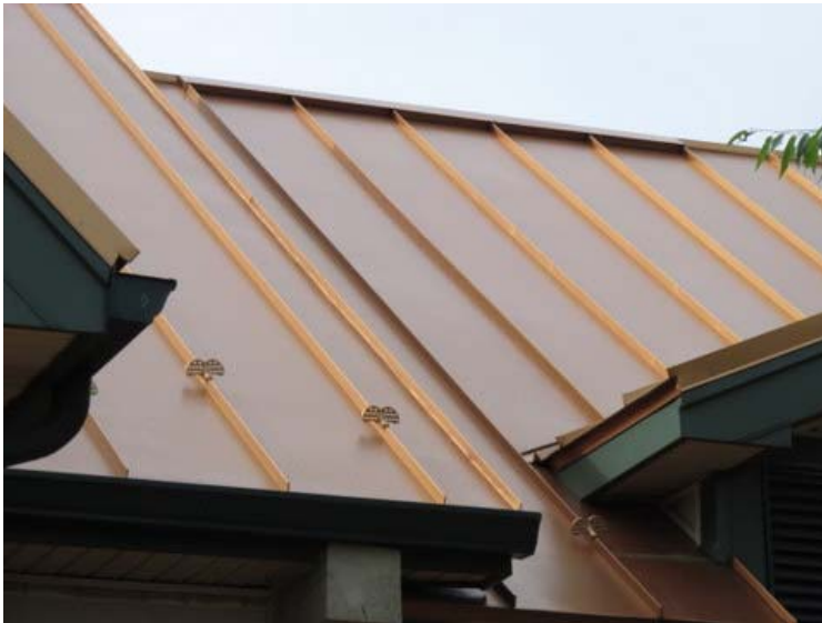
Metal standing seam roof
