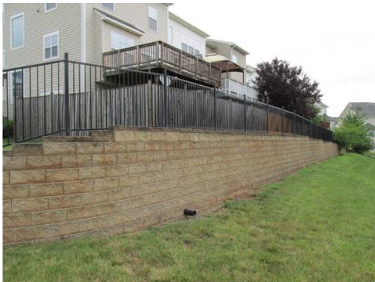
Aluminum fences atop retaining walls
