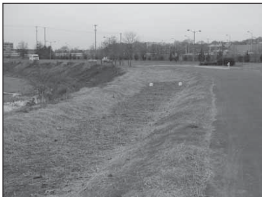
The purpose of an infiltration trench is to retain water.
