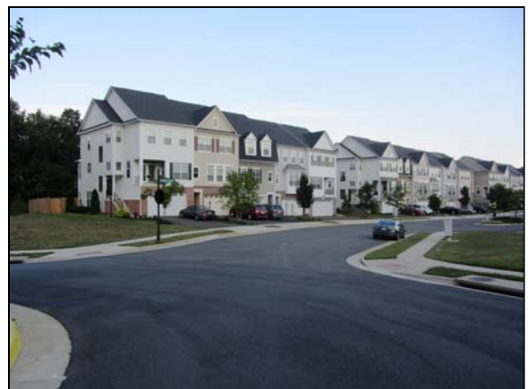
Photo #72. General view of Catbird at the assumed dividing line between publicly owned pavement and the pavement that is the responsibility of the Association.
