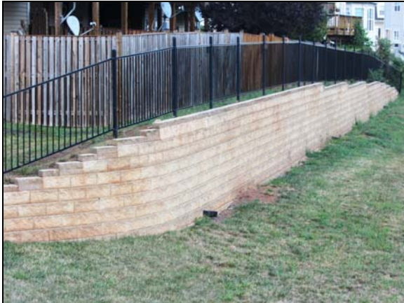
Photo #67. General view of Retaining Wall #5 located behind 14181-14203 Catbird Drive.
