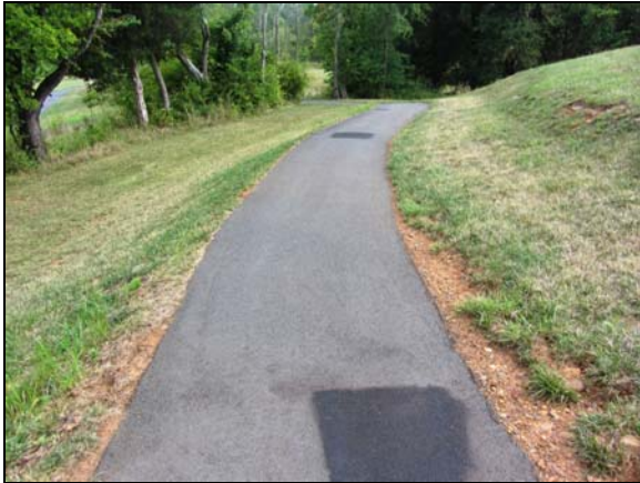
Photo #19. General view of the asphalt trail east of the swimming pool.
