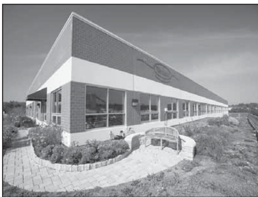
Intensive green roofs, applied on sturdier roofing systems, can accommodate paths, perennial plants, and other amenities.
