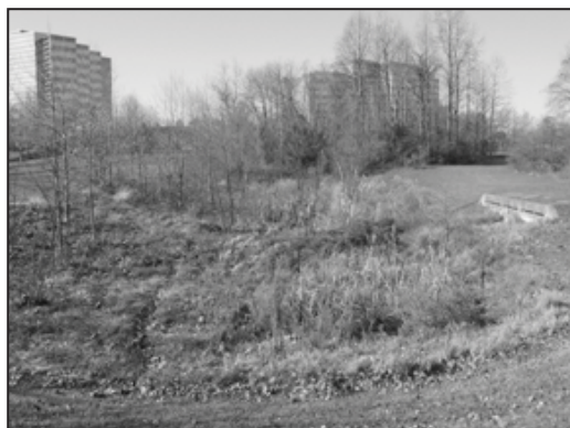
Extended detention wetland basins, or two-stage detention ponds, incorporate a shallow marsh or wetland to increase pollutant removal.
