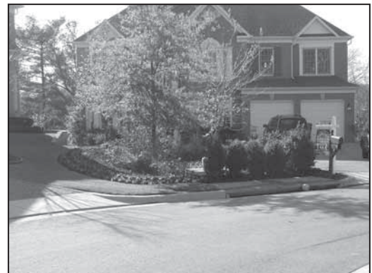
Bioretention facilities intercept stormwater runoff and use plants and soil layers to remove pollutants.
