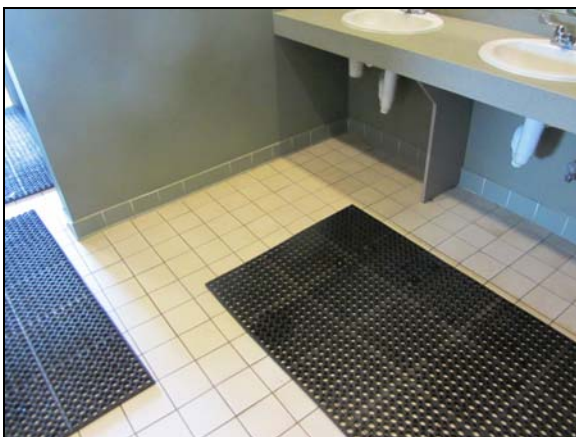
Photo #29. Typical interior finishes at the Community Center.
