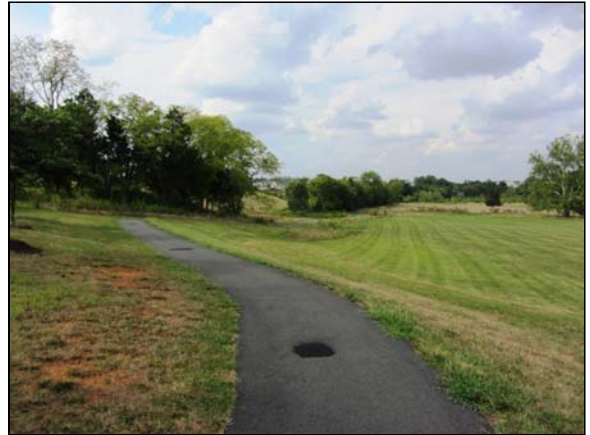
Photo #22. General view of the asphalt trail.
