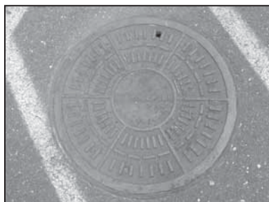
Manufactured BMP System
