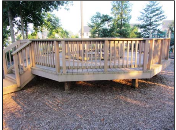
Photo #110. Deck in the Peacock Park Tot Lot area.
