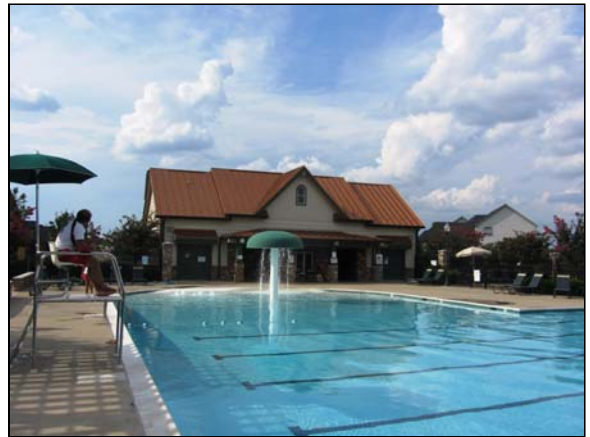
Photo #40. General view of the rear of the Community Center.
