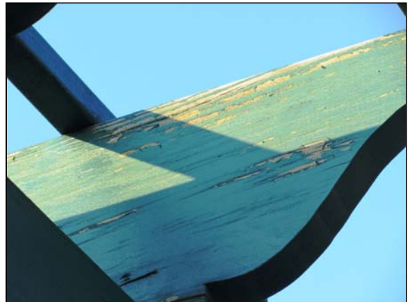
Photo #100. Detailed view of wood trellis at the sitting area south of Yellow Hammer.
