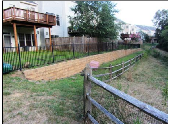
Photo #74. General view of Retaining Wall #4 located behind 14153-14163 Catbird Drive.
