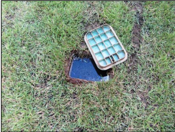
Photo #51. Irrigation vault at the northwest corner of the Community Center.
