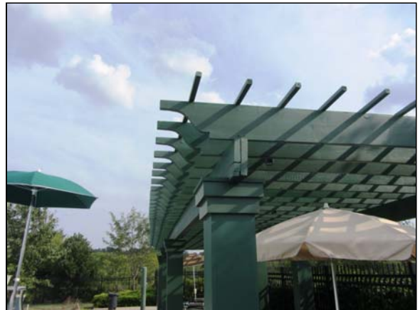
Photo #38. Trellis on the pool deck.
