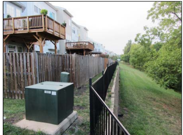
Photo #88. General view of Retaining Wall #1 located behind 14136-14146 Catbird Drive.
