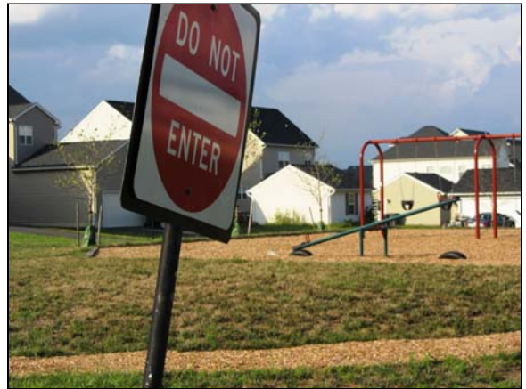
Photo #64. Typical minor damage to signage.
