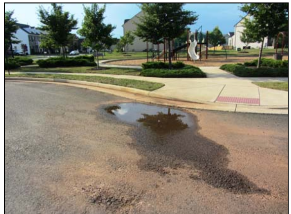
Photo #54. Asphalt pavement installation at the Community Center is not complete and silt control is still in place.
