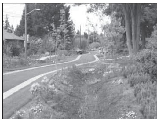
Vegetated swales serve a water quality purpose by trapping particulate matter in the vegetative groundcover.
