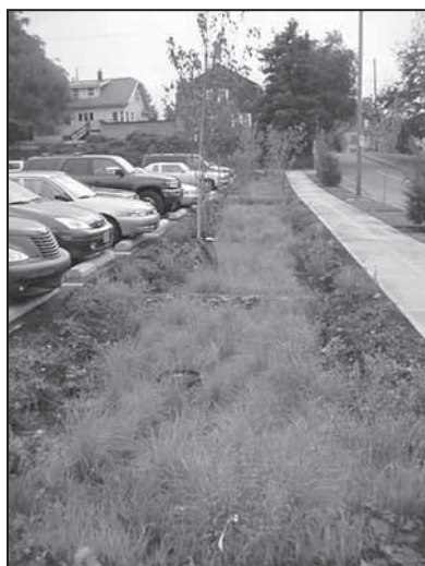
Vegetated swales are often located along roadways, parking lots, and other impervious areas.
