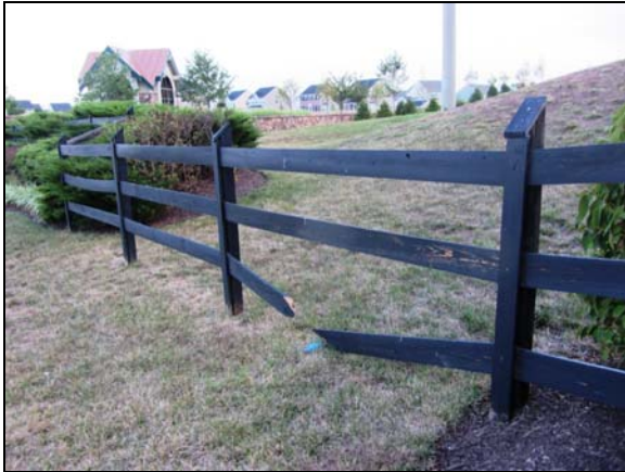
Photo #93. Damaged fence north of the Rollins Ford and Yellow Hammer entrance to the community.
