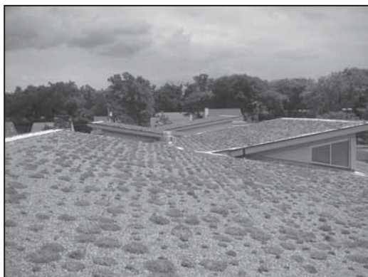
Extensive green roofs employ succulent low-growing plant species, such as sedums.
