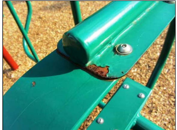
Photo #56. Failed paint system on the tot lot equipment, South Tot Lot.
