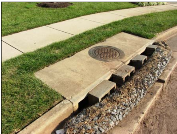
Photo #53. Asphalt pavement installation at the Community Center is not complete and silt control is still in place.
