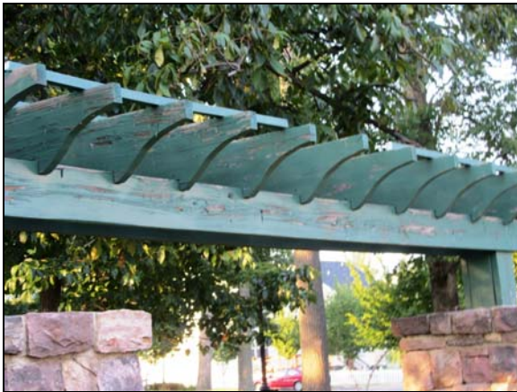
Photo #105. Typical trellis installation at the entrances to Peacock Park.
