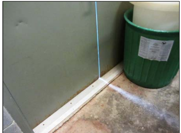
Photo #46. Minor rusting of the doors at the Community Center.
