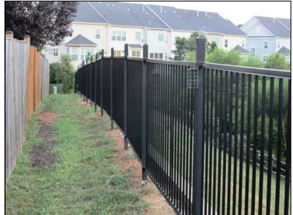
Photo #68. Excellent grading behind Retaining Wall #5.
