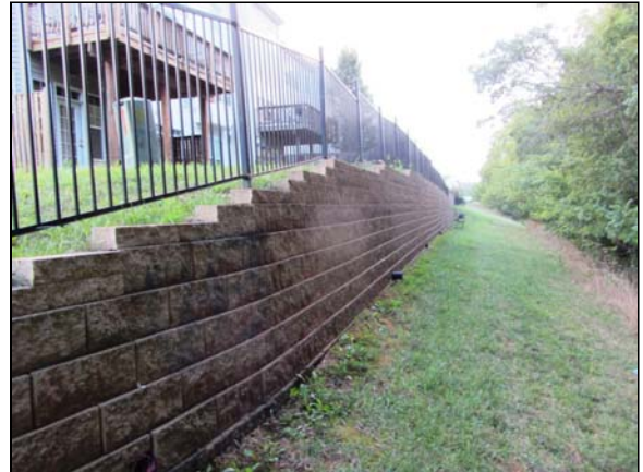
Photo #86. General view of Retaining Wall #2 located behind 14122-14132 Catbird Drive.
