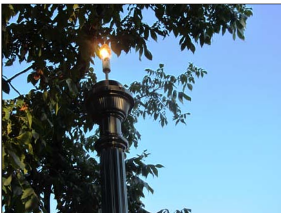
Photo #107. Damaged light fixture on the south side of Piedmont Park near the entrance.
