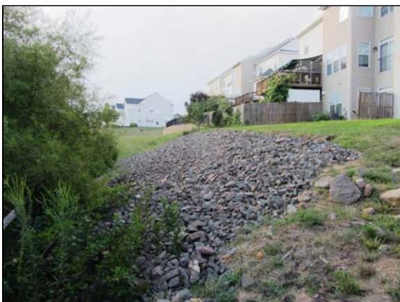
Photo #71. Rip rap installed on a steep slope in the vicinity of 14181 Catbird.
