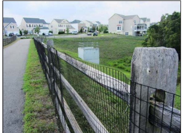
Photo #80. Detailed view of the fence surrounding the dry pond south and west of Catbird Drive.
