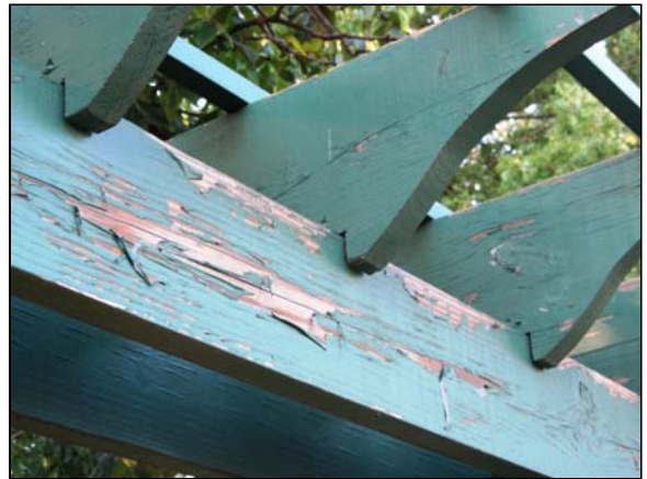
Photo #106. Detailed view of the trellis installation at the south entrance to Peacock Park.
