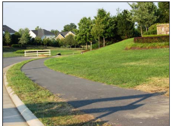
Photo #114. Asphalt trail installed along Rollins Ford.
