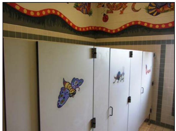
Photo #30. Typical interior finishes at the Community Center.
