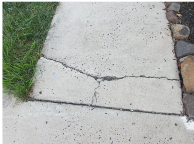
Sidewalk cracks
