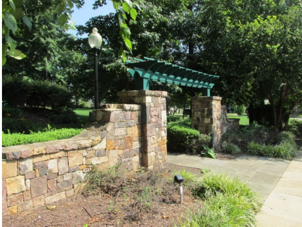
Arbor and masonry wall at Parula Park
