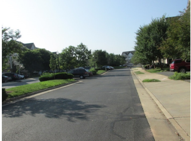
Townhome pavement overview
