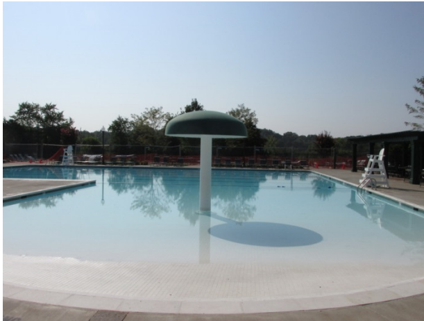
Main pool overview
