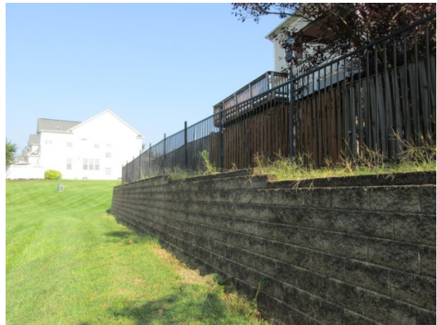
Masonry retaining wall
