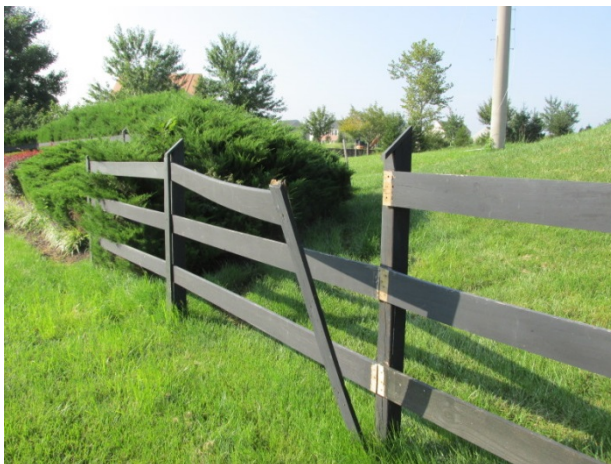
Fence displacement
