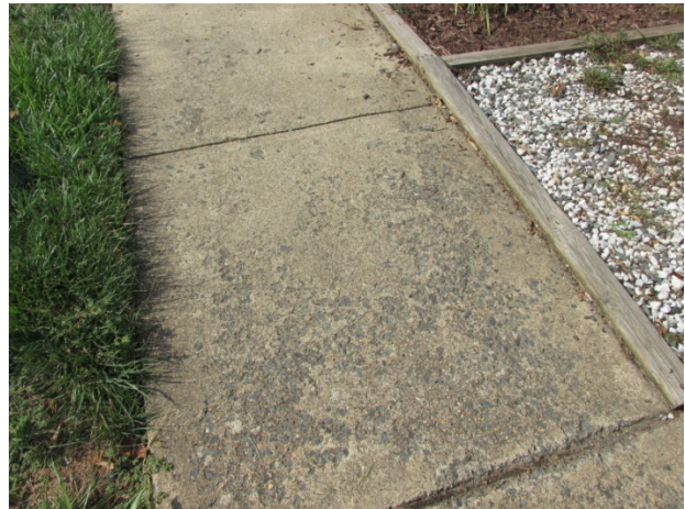
Sidewalk spall
