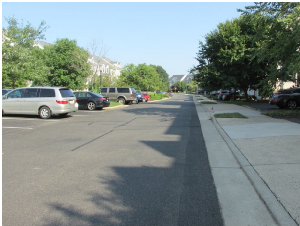
Townhome pavement overview
