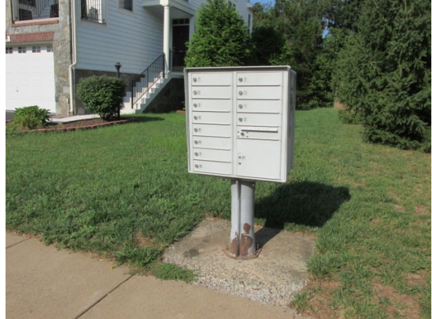
Mailbox station (Note: Finish deterioration evident)
