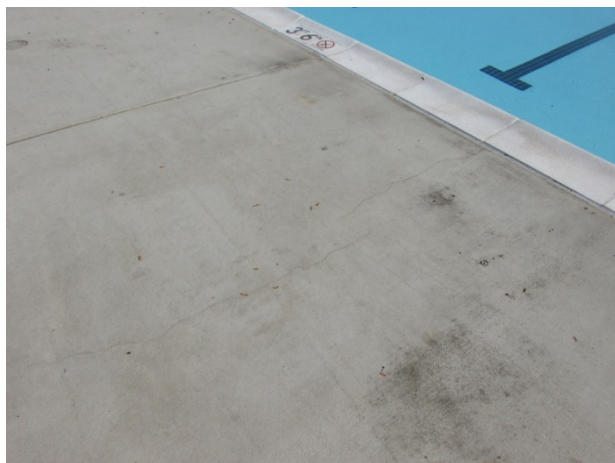
Deck crack
