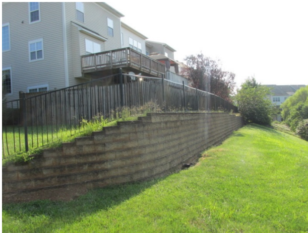
Masonry retaining wall
