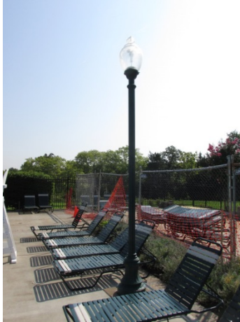
Light pole and fixture
