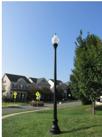
Light pole and fixture
