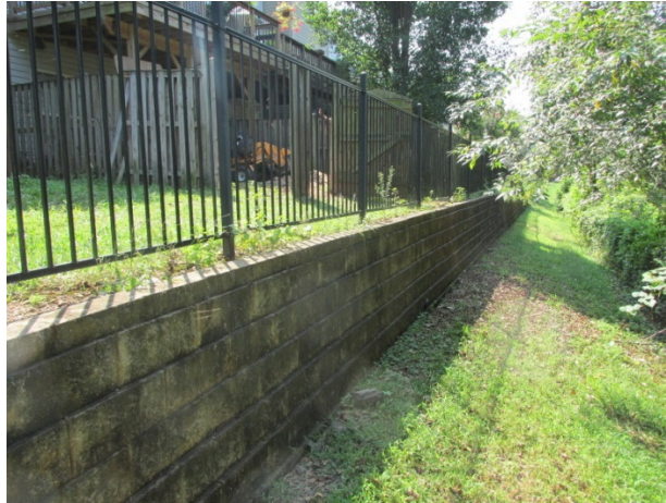
Masonry retaining wall
