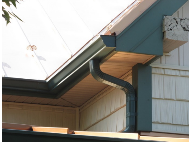
Aluminum gutter and downspout assembly
