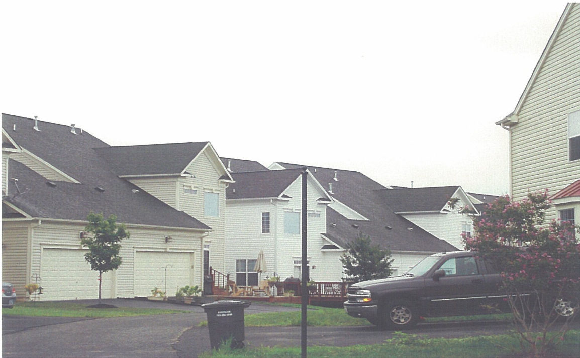
The sign is missing from the post at the alley entrance on Woodpecker Court.
